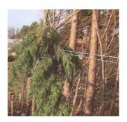
The Event: A Certificated and Authorised work team reducing a cypress hedge with the circuit Live. The operator of the MEWP used a Silky saw to cut a step cut into the stem. He attempted t to lift the stem by holding it and moving the MEWP bucket. It got caught up and he lost his grip and it fell onto the LV line causing Phase to Phase contact and a loss of supply. There were no injuries.
