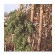
The Event: A Certificated and Authorised work team reducing a cypress hedge with the circuit Live. The operator of the MEWP used a Sliky saw to cut a step cut into the stem. He attempted t to lift the stem by holding it and moving the MEWP bucket. It got caught up and he lost his grip and it fell onto the LV line causing Phase to Phase contact and a loss of supply. There were no injuries.
